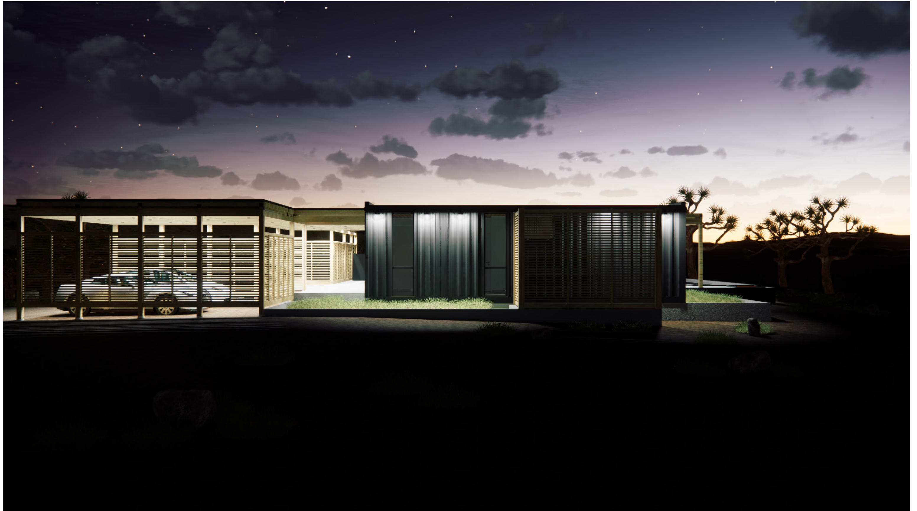
East Exterior (Night)
