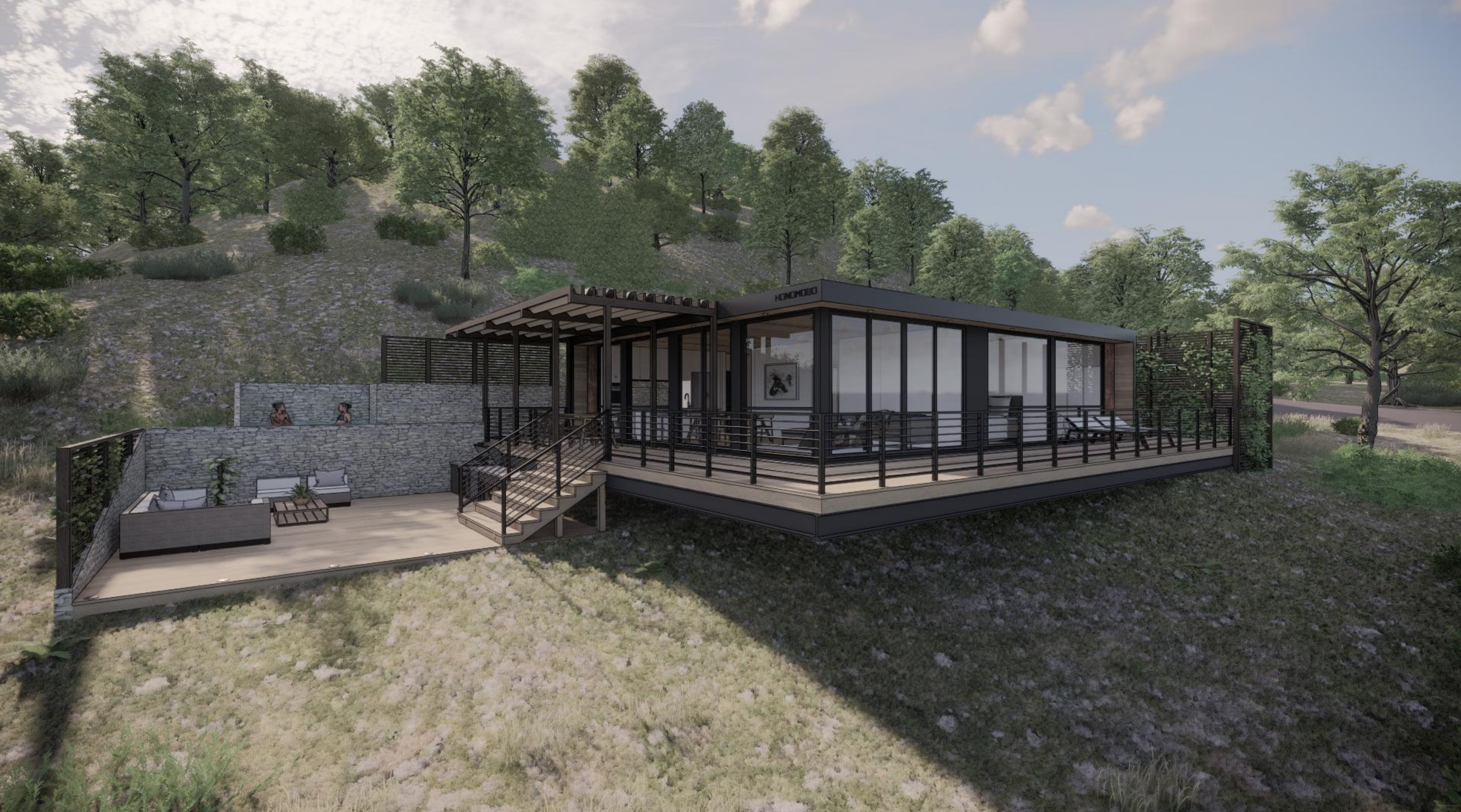
North East Exterior
