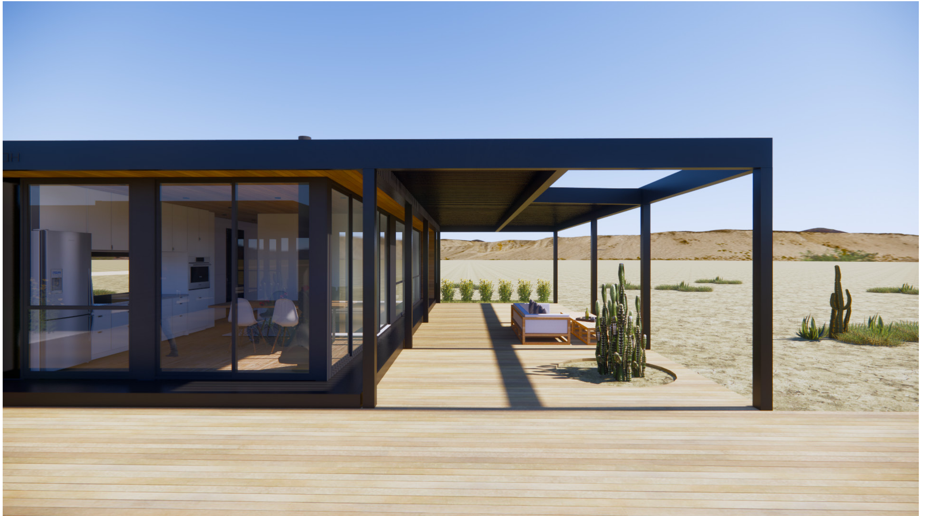
The North View of HO2
